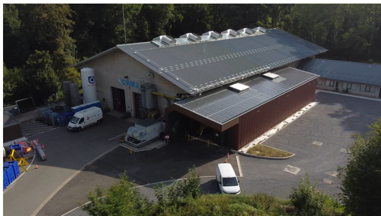
Green Electricity: PV steel roof
