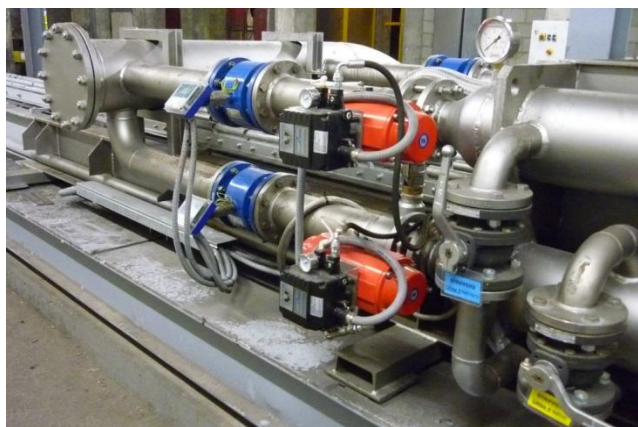
Figure 11: Balancing valves with flowmeters for slit-rolling
