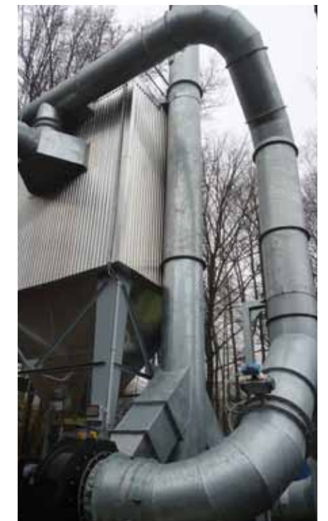
■ A new bag filter to treat the fumes of several reactors
