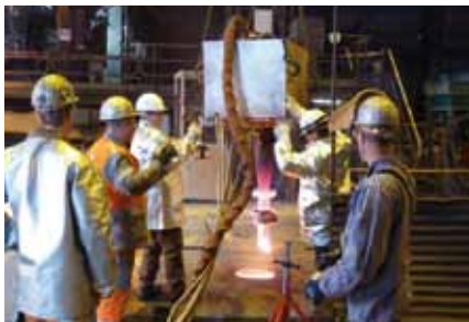
■ Installation of the LIBS unit in the Blast Furnace hot metal runner
