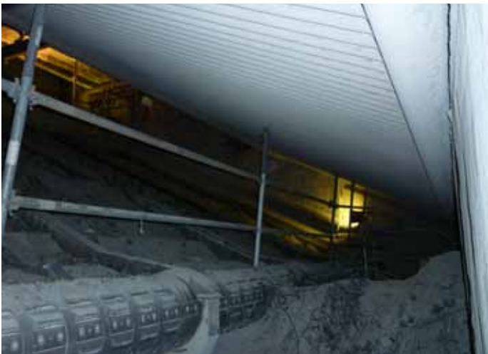
Fig. 46 Exchanger tubes corrosion in an urban incinerator
