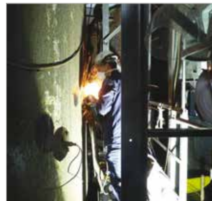
Installation of strain gauges onto the BF shell
